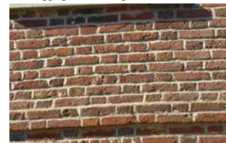
Figure 33: example of Flemish bond brickwork, common within the Character Area
