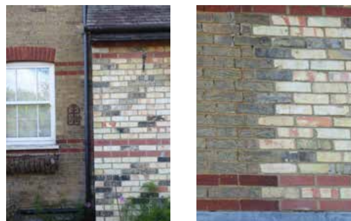
Figure 88: Poorly matched, bright modern brick, can contrast poorly next to original buildings if not well considered
