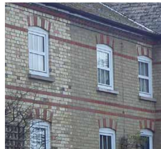
Figure 52: An example of where modern uPVC windows have been installed to replace wooden sashes
