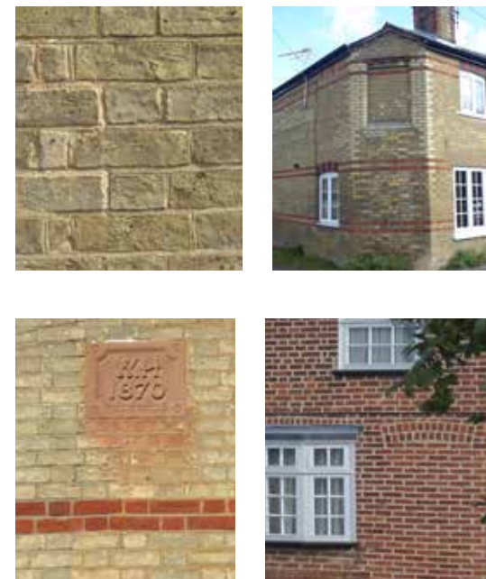
Figure 70: Examples of brickwork within the Character Area
