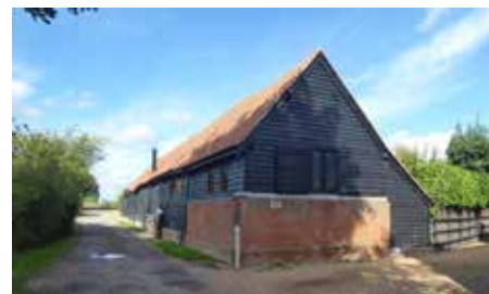
Figure 49: Barn at Burge End Farmhouse
