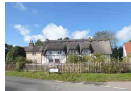
Figure 31: 4-6 Walnut Tree Road
