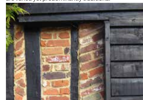
Figure 38: An example of exposed timber framing and brick nogging, found throughout the Character Area
