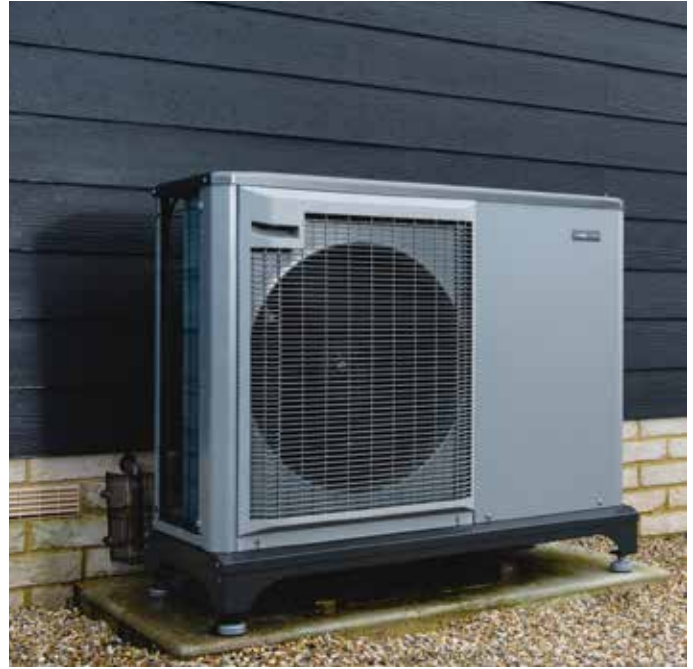
Example Air Source Heat Pump
